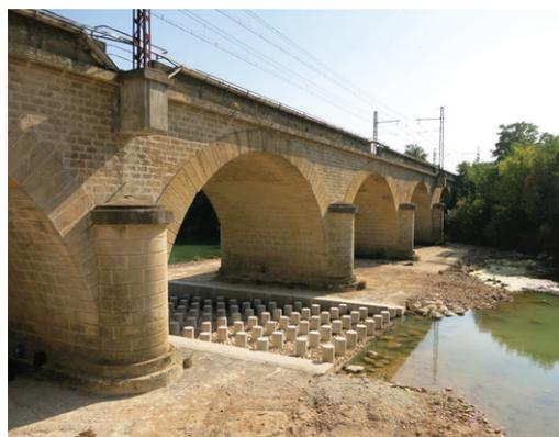
Riprap fishway at sill level under the Vidoule Bridge in Gallargues le Montueux
